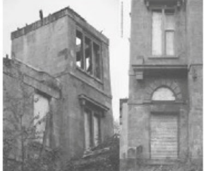
east/north sides of the tower top
