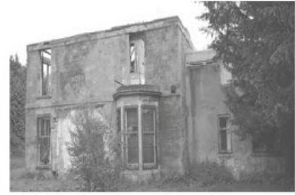
south elevation with a smaller ground floor bay window
